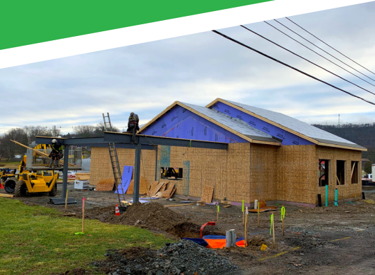
Progress on C&N's new Towanda office
